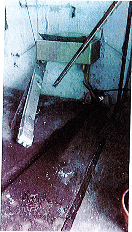
Image 6. Belfast sink, Channel, sluice, and remnants of panel fixings
