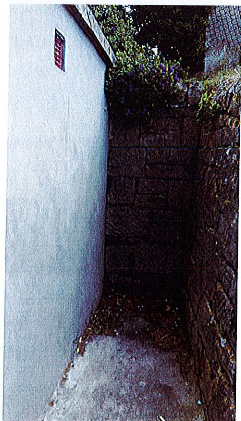
Image 3. Side wall to retaining wall of Gardens
