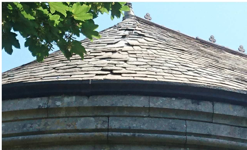
North facing roof tiles
