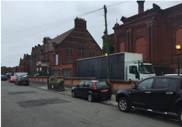
Hartley's Village, Factory Complex
